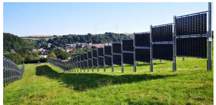
Figure 4: Sample use of vertical bifacial PV panels by Next2Sun
