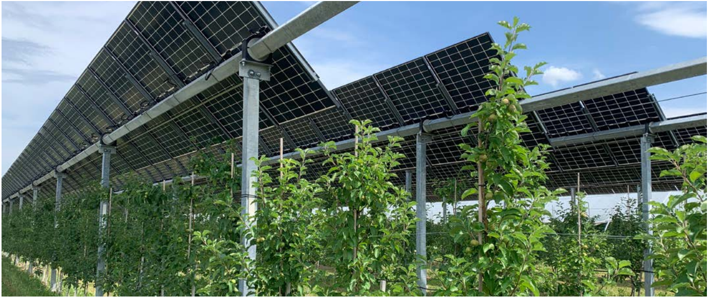
Figure 8: Bifacial tracking system by Intech GmbH & Co. KG above fruit trees
