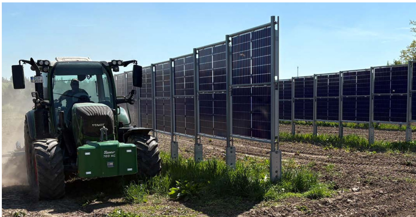
Figure 9: Sample vertical interspace system at Energiepark Neusaß II. Image: Gerd Herold
